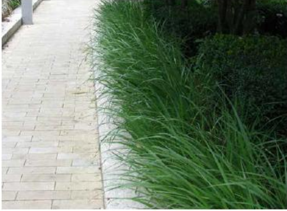
Stone kerb edging to planting. Yorkstone paving
